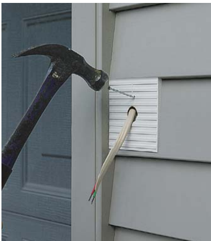
Can be nailed or screwed in place
